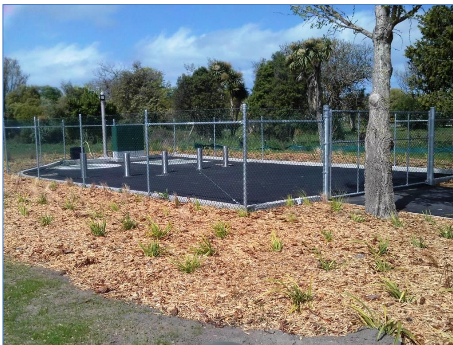
Photo of existing wastewater pump station on Hilton Street
